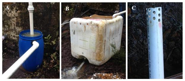
**Figure 4.** A. Image of diversion well with inlet piping AMD and an outlet allowing flow into settling pond. B. Image of IBC used as a settling pond. Water from well piped into top of settling pond, treated water outflow at base into Cannel Creek. C. Image of perforated 50 mm inlet pipe into diversion well.
